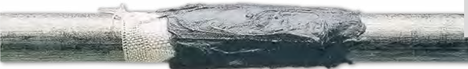
Emergency repair of a water pipe
